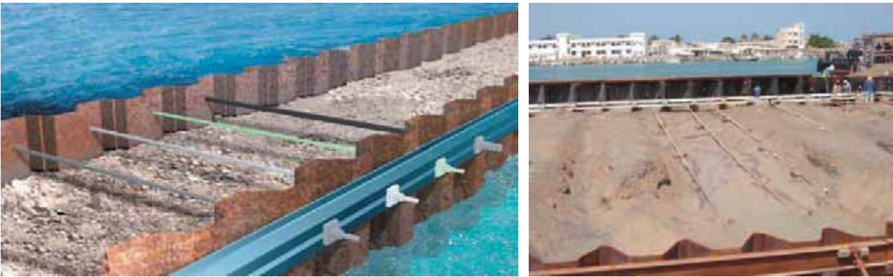
Marine works - Ras al kaimah port Phase 1, UAE
