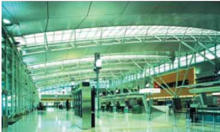
Qantas Departure Hall Project in Sydney, using CT Bars
